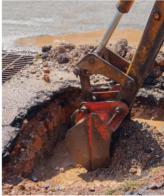
Figure 6: Another Common Cause of Fiber Breaks
