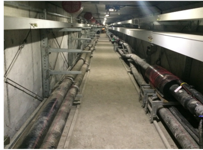
Fig. 6. 220kV Cables in Tunnel requiring On-line PD measurement.
