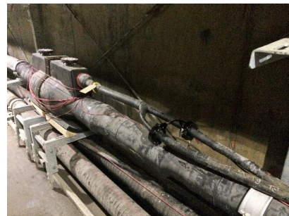
Fig. 7. RFCT sensor on earthing of 220kV Cables in Tunnel.
