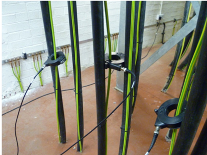
Fig. 2. RFCTs installed on the earth conductor of single-core cables.
