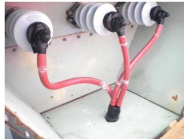
Fig. 1. Partial discharge caused by incorrect installation found on a cable termination using non-intrusive PD instrument.
