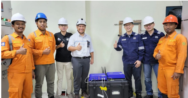
Figure 1: EA Technology engineers and onsite operators from PLN UPT Bali.
