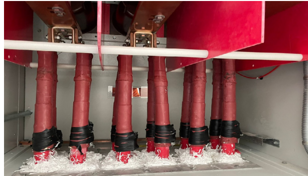
Figure 6: AFTER remedial action - anti-tracking sheds were removed.
