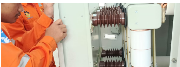
Figure 2: Onsite operators opening up the identified area.
