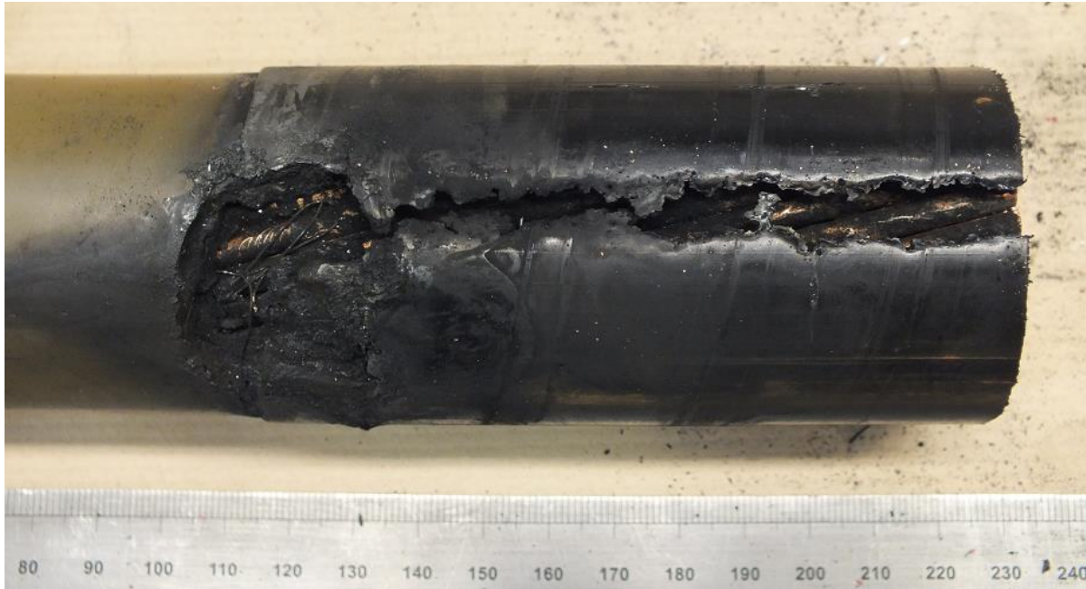
Figure 8. Linear arcing damage in the cable
