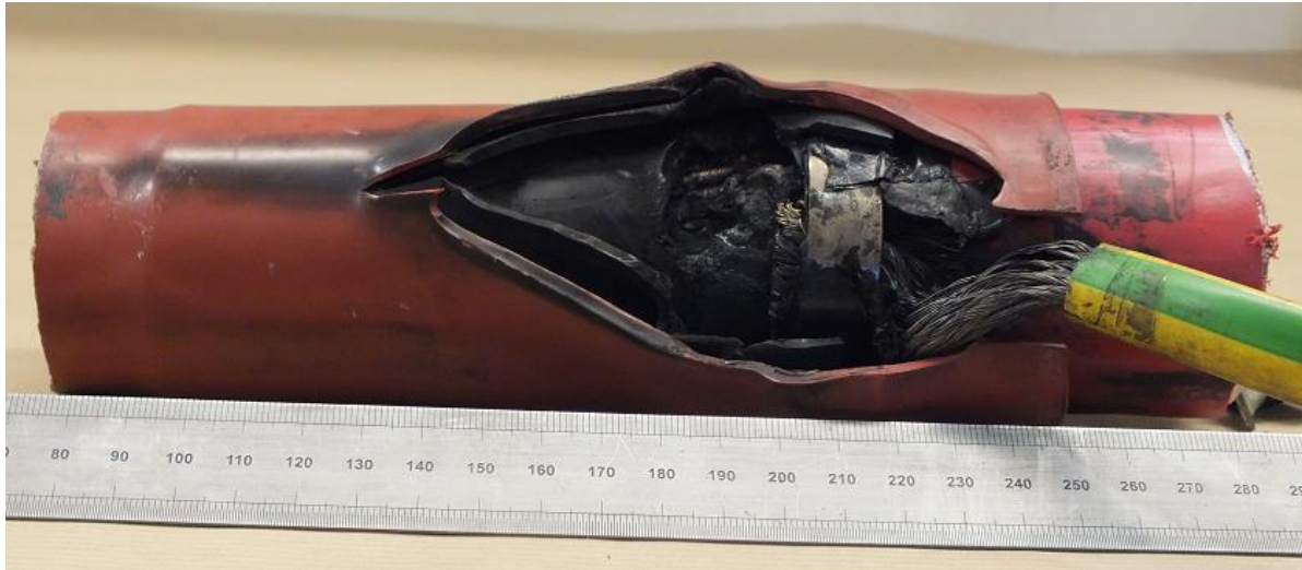
Figure 2. View of the fault hole in the failed termination
