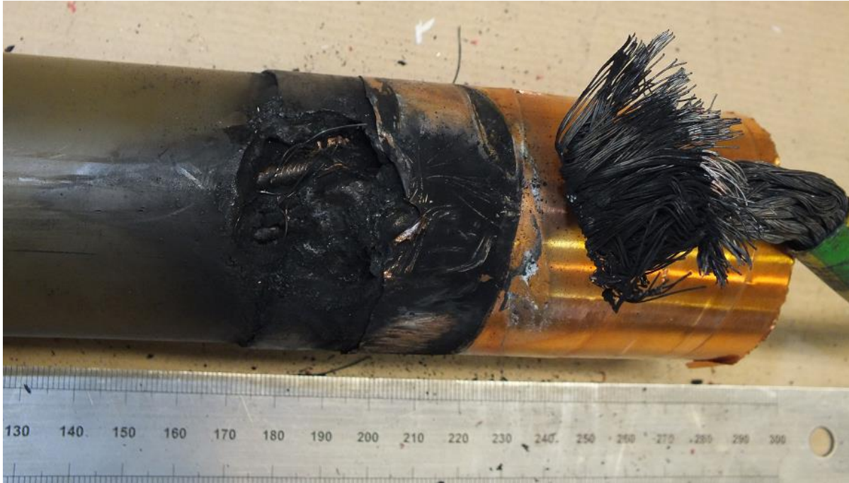
Figure 7. Contact area between copper tape and earth lead blackened, but not arc damaged. Arcing damage on the tape is above the roll spring position.
