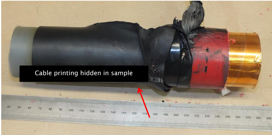
Figure 4. Failed termination: stress control tube creased next to fault damage
