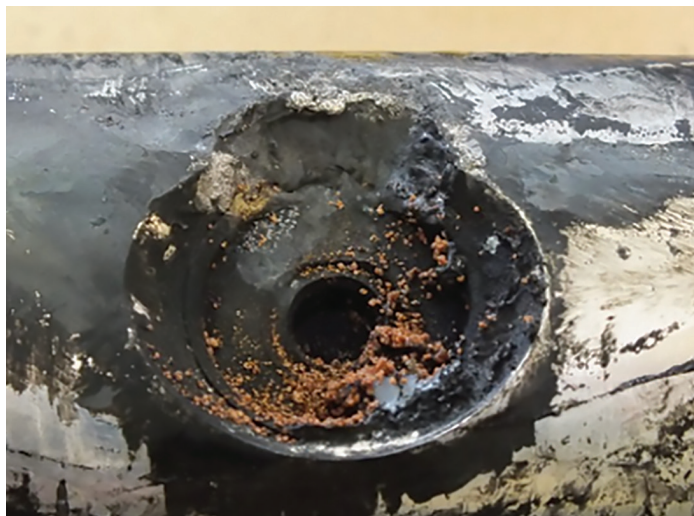
Figure 13: Failure Location on 33KV XLPE Joint
