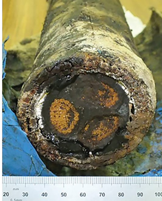
Figure 14: Failed PILC Cable
