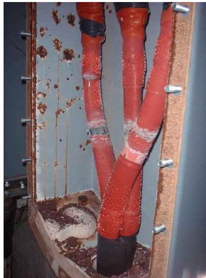
Figure 5 - Discharge on a circuit breaker caused by high humidity and a design flaw
