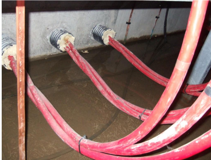
Figure 3 – Flooded cable trench
