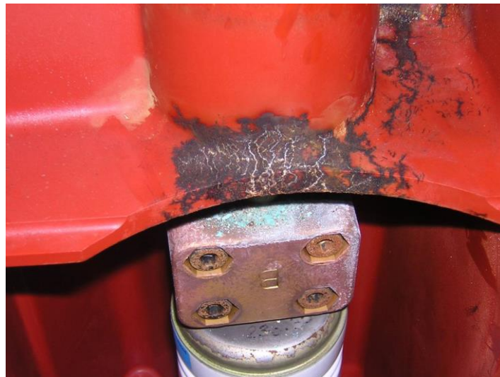
Figure 5 - Discharge on a circuit breaker caused by high humidity and a design flaw
