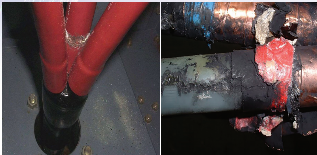
Partial Discharge Damage at Field Terminations as a Result of Poor Workmanship
