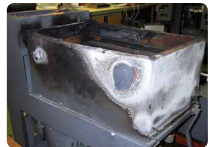
Explosion in 3.3kV circuit breaker
