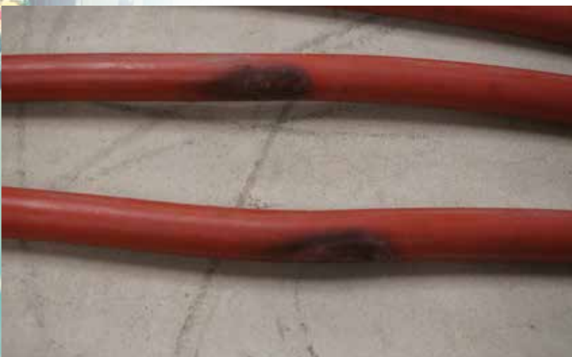
Figure 6: Damaged PT Cables
