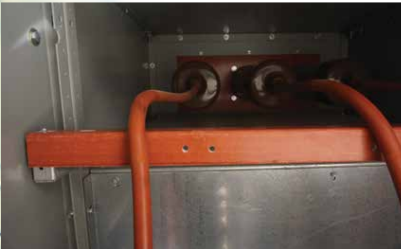
Figure 5: Improper Cable Installation
