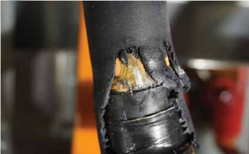
Figure 4: Damaged Cable Termination
