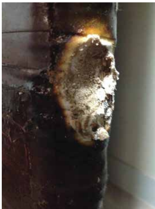
Figure 3: Close-Up of Damage on Edge of Busbar
