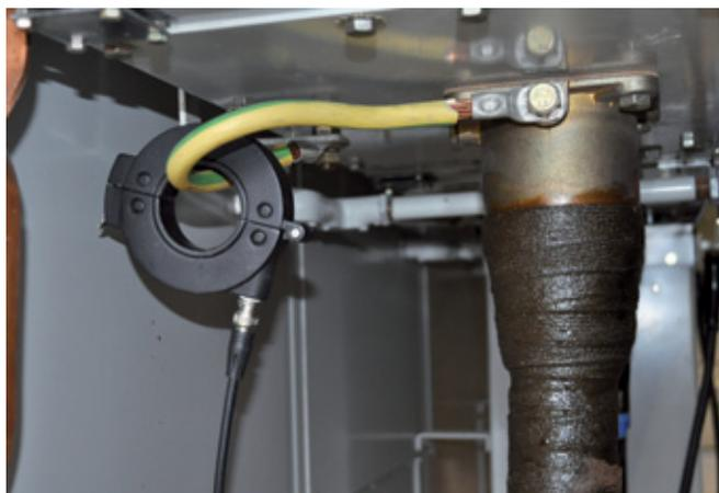
**Figure 2** RFCTs installed on the earth conductor of single-core cables.
