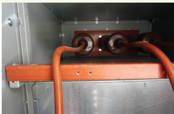
Figure 6: Improperly Installed PT Cables
