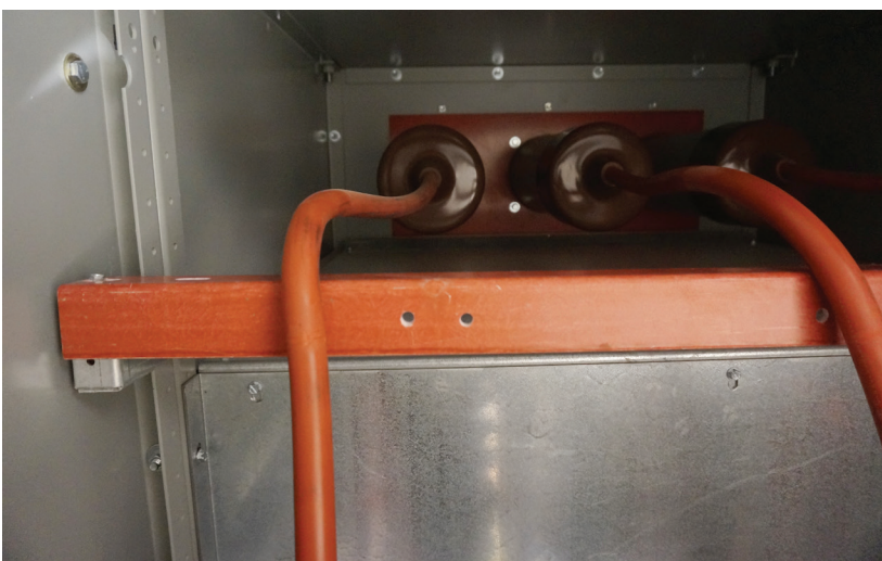
Figure 6a: Geometrically Induced PD
