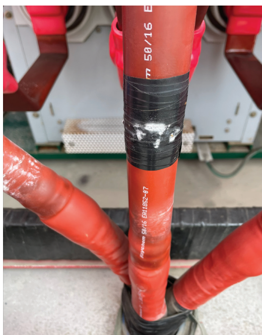
Figure 5: Phase ID Tape Causing PD
