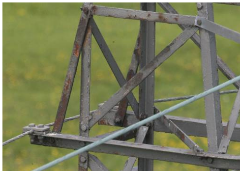
Figure 3: Steelwork and degradation of protective coating.
