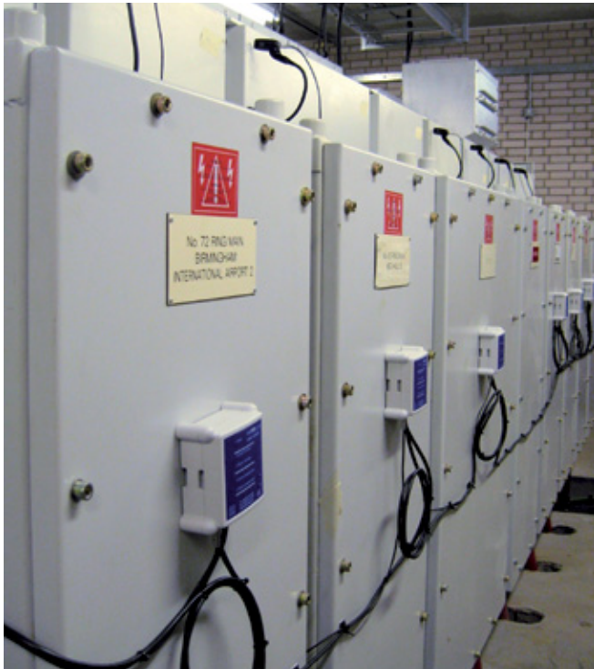
Figure 2 Example of a continuous online monitoring system for partial discharge in MV switchgear
