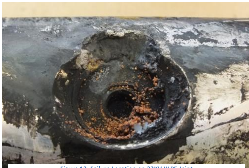
Figure 13: Failure Location on 33KV XLPE Joint
