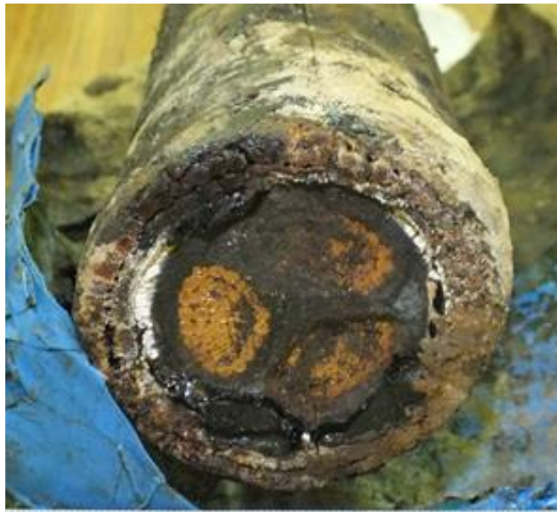
Figure 14: Failed PILC cable
