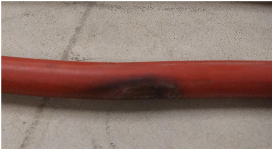
FIGURE 8: PD damage to a PT cable.
