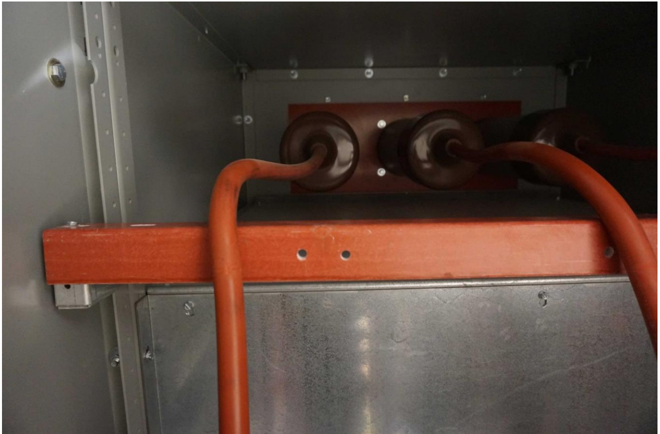
FIGURE 6: Improperly installed PT cables.
