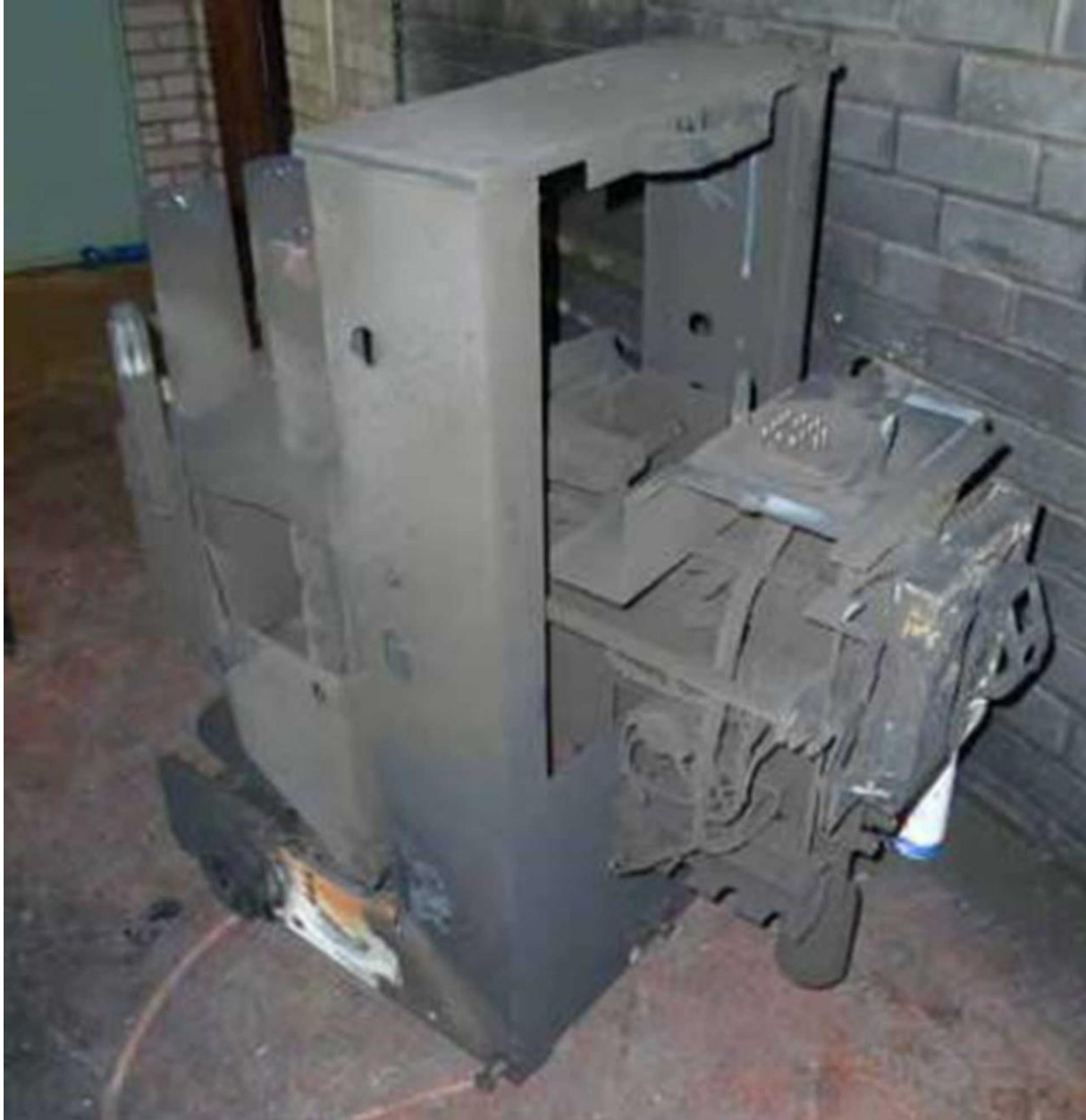
FIGURE 1: As a result of inaction, the switchgear at a U.K. utility experienced a catastrophic failure.
