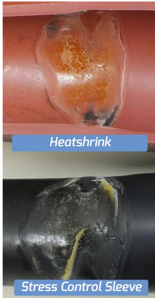
FIGURE 5: The root cause was identified to be an incorrect gap between the XLPE insulation and the connector being only 1 mm instead of the recommended 5 mm, preventing the yellow mastic from filling the gap properly and leaving a void that led to the elevated electrical stress responsible for the detected PD.
