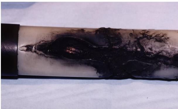
Damage from flashover to screen
