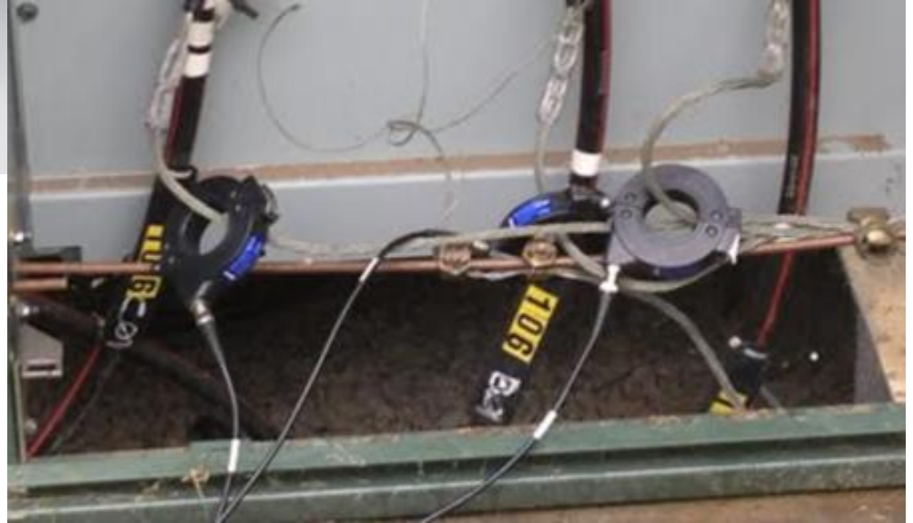
RFCT Installed on Ground Straps
