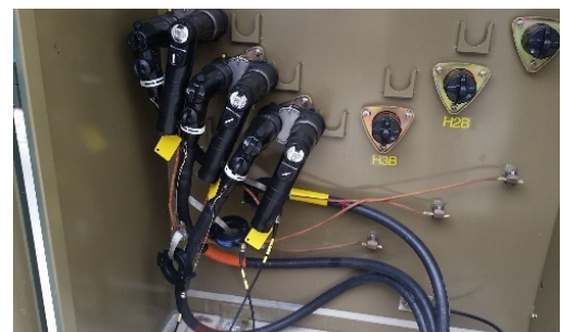
Cable termination in metal-clad switchgear
