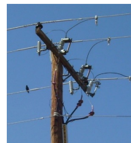
Cable termination on riser pole
