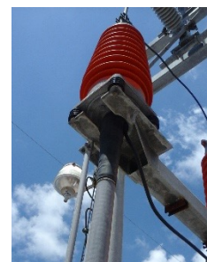
Cable termination in 69KV switchyard
