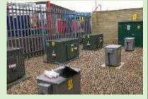
units the use of the EES devices for peak shaving, solar power absorption, voltage support, phase balancing and aggregated demand reduction was demonstrated.
