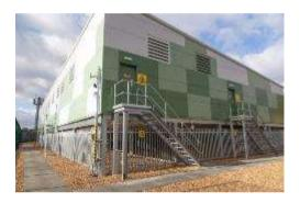
Figure 8.2: 6MW/10MWh EES System (UKPN)
