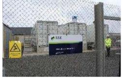
Figure 8.3: 2MW/500kWh EES System (SSEPD) - Containerised
