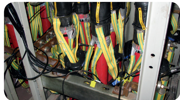
Figure 2 RFCT Installation
