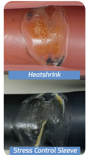
Figure 4 Evidence of PD activity
