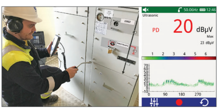
An UltraTEV Plus 2 was used to pinpoint the problem and measure PD activity in detail.
