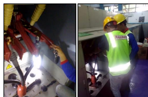
Fig.6. Replacing Cable Terminations Canda Feeder
