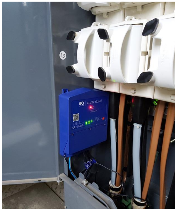
ALVIN Guard Installation
