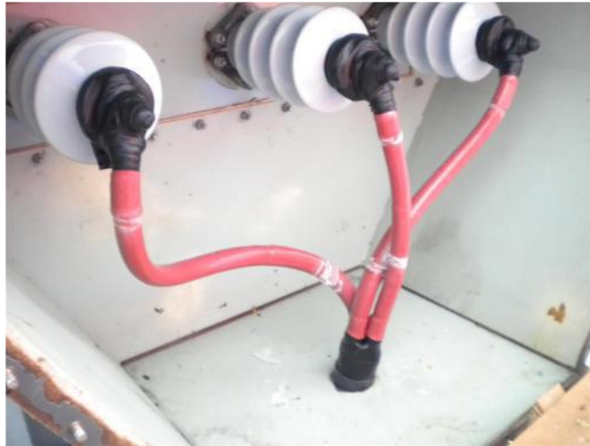
Partial Discharge damage on Cable Terminations
