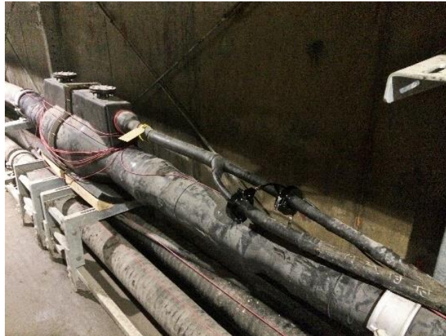
RFCT sensors on earthing of 220kV Cables in Tunnel.
