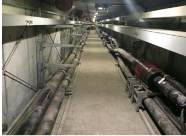
220kV Cables in Tunnel requiring On-line PD measurement.
