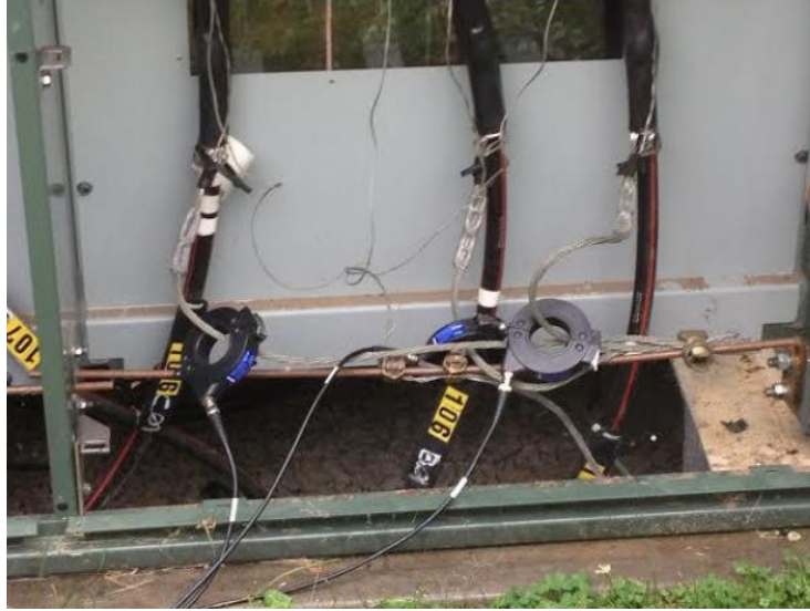
Example of Radio Frequency Current Transformers installed on Sheath Grounds
