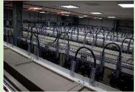
**Project Description:** This project demonstrates the operation of a 1MW/3MWh VRLA Pb-Acid battery, deployed as part of a wider Smart Grid trial. The system is intended to inform the strategy to replace Lerwick Power Station, and will provide peak shaving, frequency response (on Shetland’s island network), voltage support and allow the connection of additional renewable generation.
