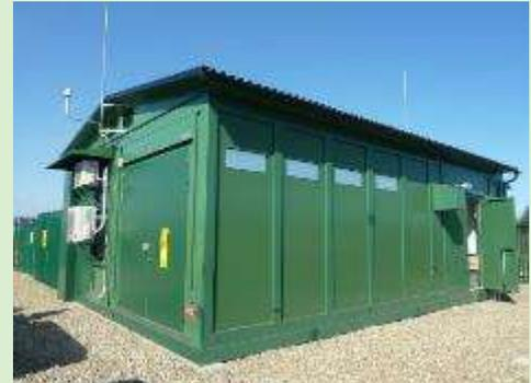
**Project Description:** This project was the first DNO battery energy storage project installed as part of the LCN Fund. The 200kW/200kWh Li-Ion system was used to carry out peak shaving, wind farm output regulation, voltage support and aggregated demand reduction.
