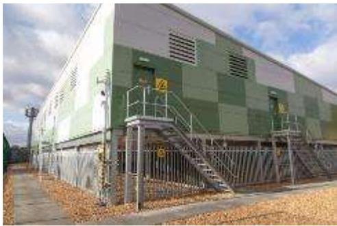
**Figure 8.2: 6MW/10MWh EES System (UKPN)**
