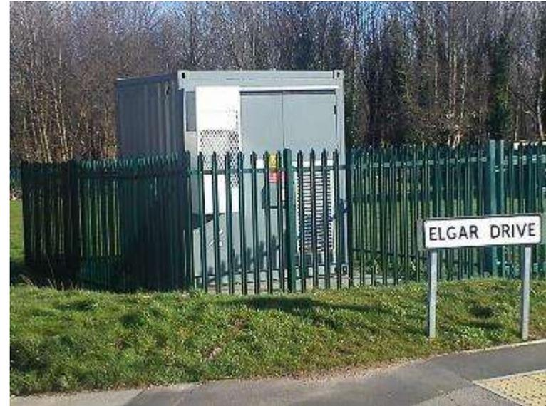
Figure 2.10: 50 kW, 100 kWh ESS in Sheffield (Source: Northern Powergrid)
