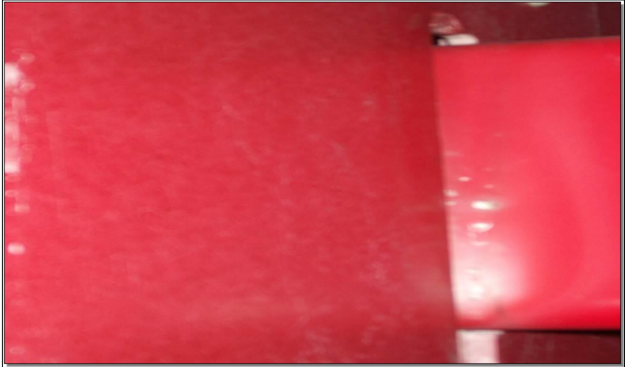
Photo 6: Insulation Emitting PD
