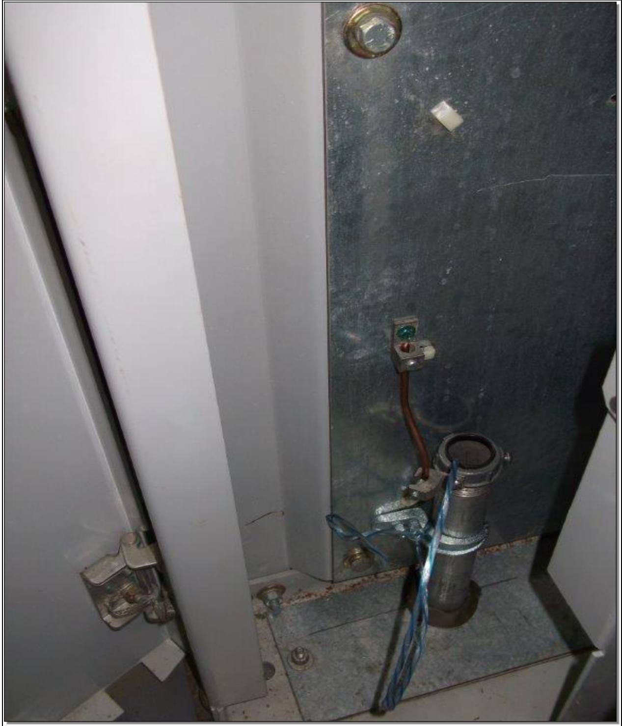
Photo 3: Conduit Penetration - Under Floor
