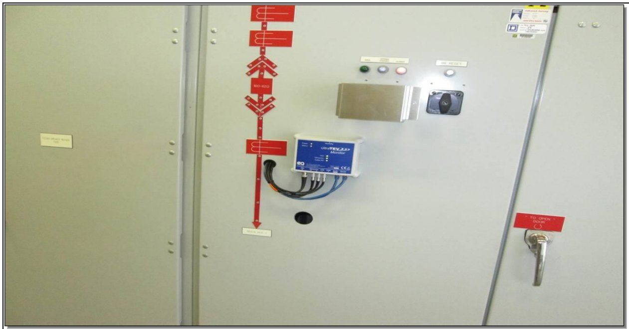
Photo 1: Node Installed on Exterior Cubicle Door
