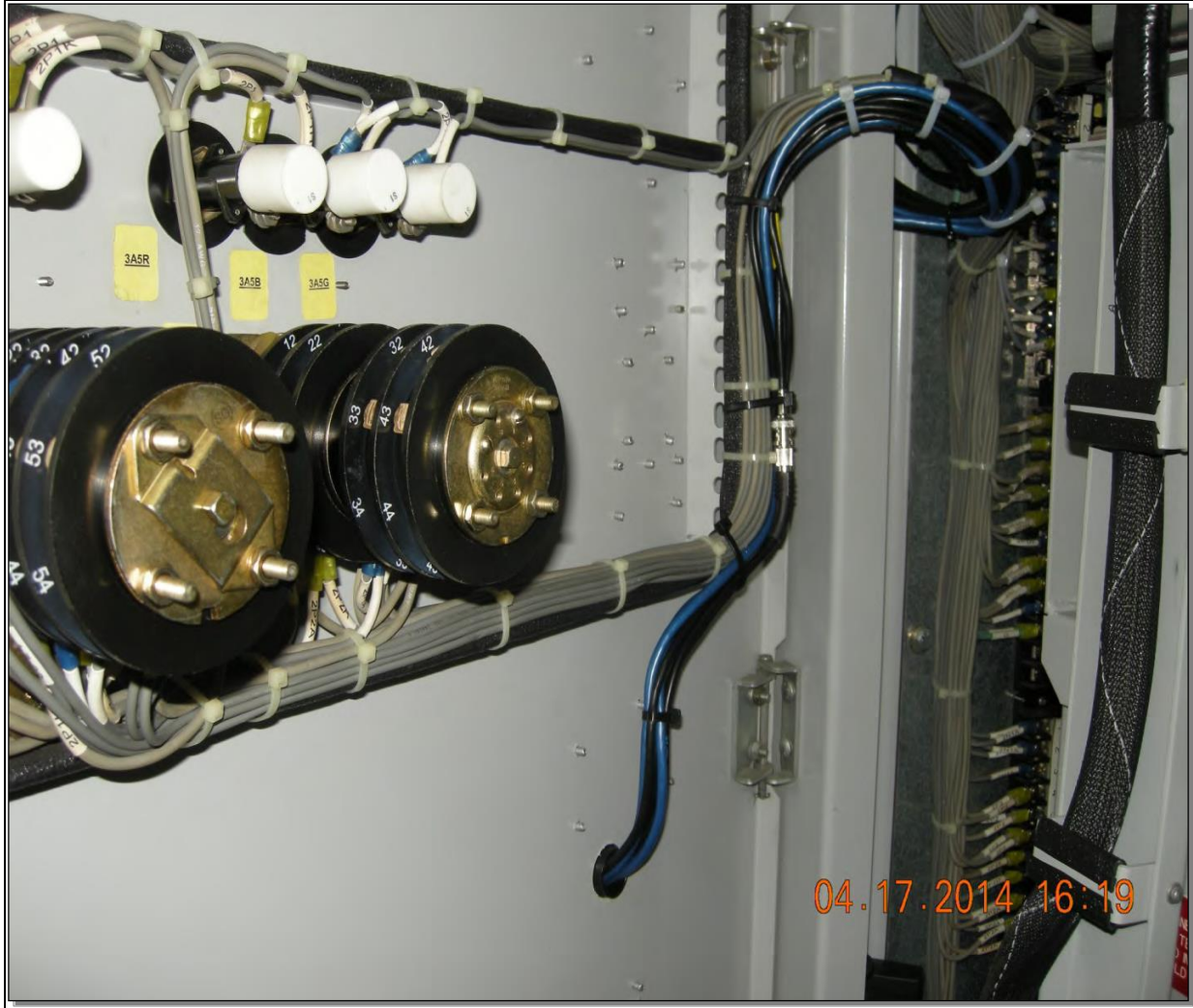
Photo 2: Cable Routing to Node through the Door
