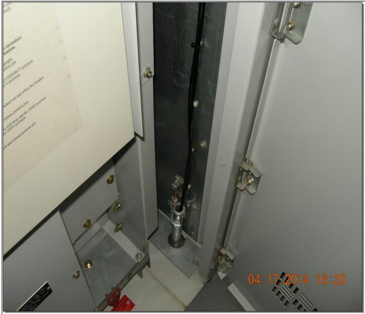
Photo 4: Cable Pulled In Underfloor Conduit
