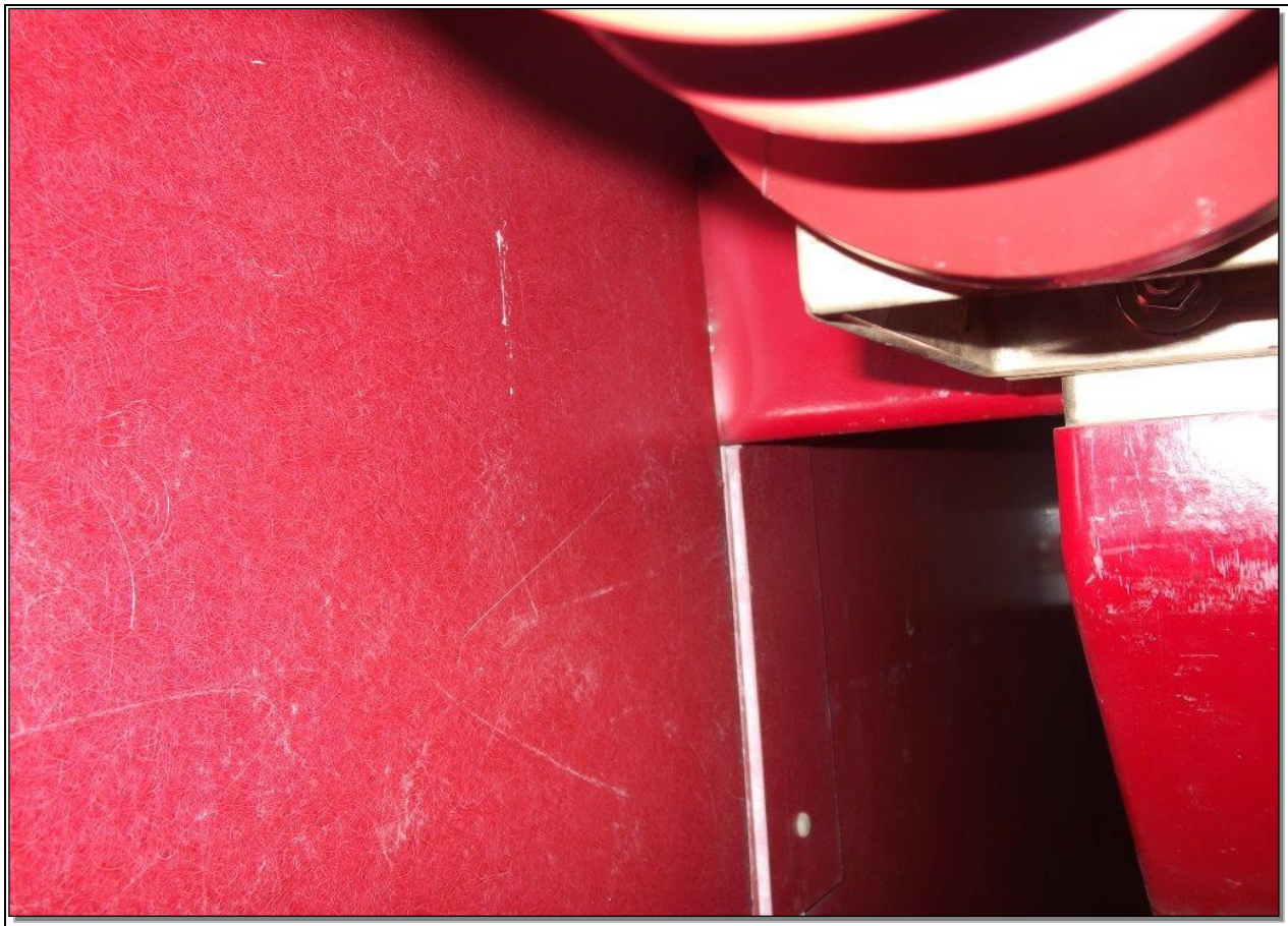
Photo 5: Insulation Emitting PD
